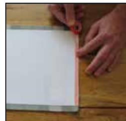
6. Apply double-sided tape to the PVC panel edge. This will be used to stick the seam.
