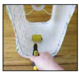
**21.** For best results use a seam roller to apply the pressure, rolling up and down the seam.
