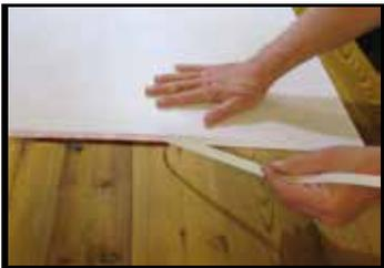
7. Carefully, to avoid fraying, remove the broken strips of PVC to leave your covering's edge.
