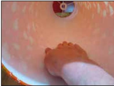
**16.** Turn over so the seam is now on a hard surface and apply firm pressure pressing the tape down with your hand.
